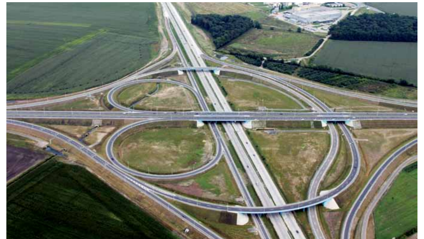
Wrocław Motorway Bypass
